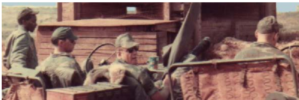
1b. Pleiku AB, Bravo-3 Bunker. Close up. 1968.
