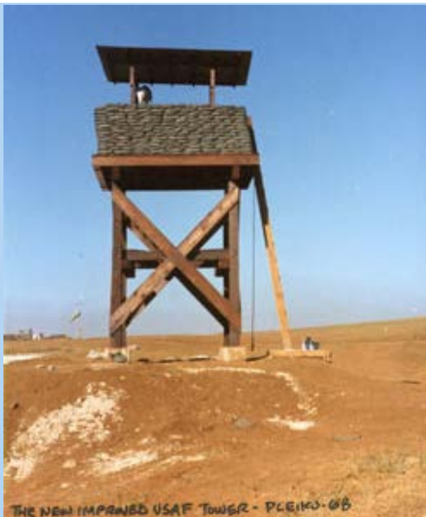
3. Pleiku AB, Perimeter Tower (new and improved). 1968.
