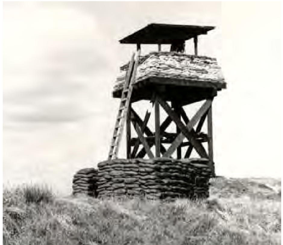
54. SP Tower Bunker-10.
