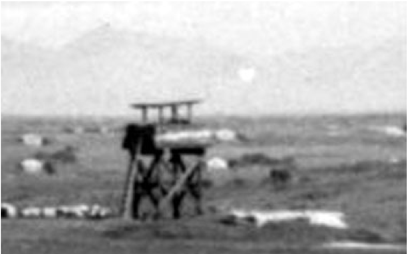
33. Pleiku Air Base, perimeter Tower, closeup.
