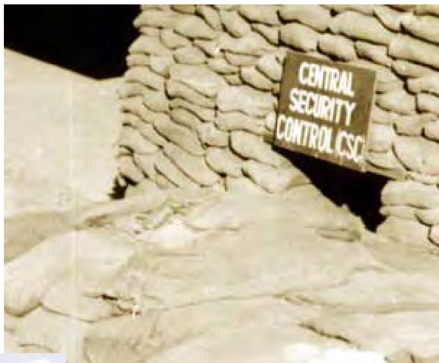
43. Right. Central Security Control (CSC).
