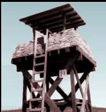
5) Perimeter New Tower #24.
