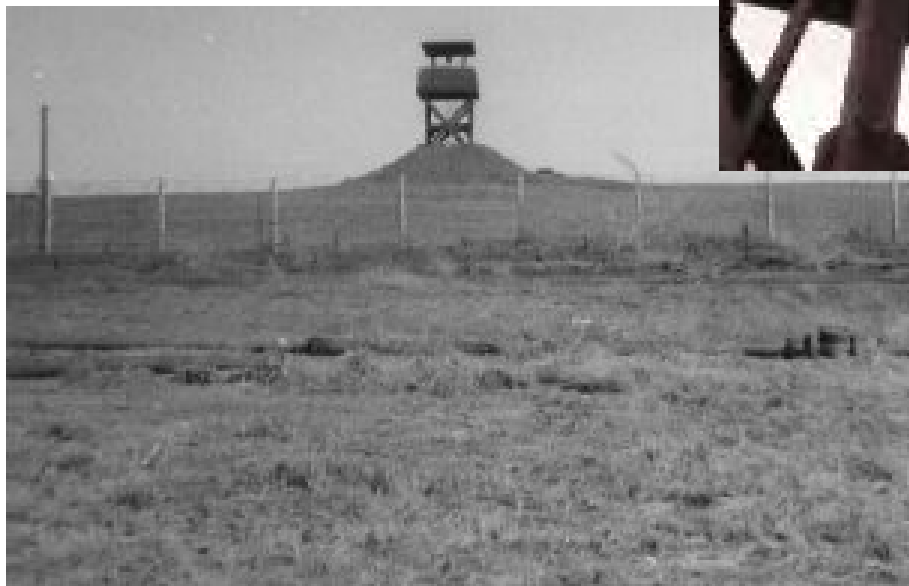
26. Left. View of Tower from Perimeter.
