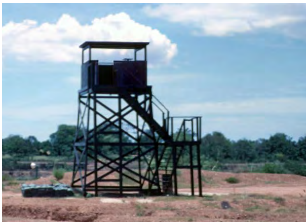
6b. Phù Cát AB, Perimeter Tower and Bunker. Photo by David Hayes, LM 462, CRB, 12th SPS; PC, 37th APS, 1967-1968.
