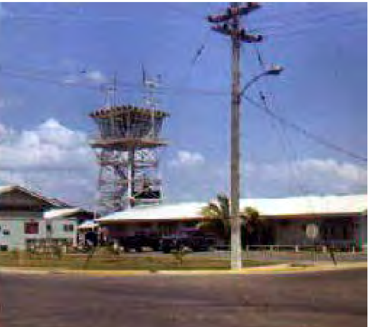
05. (above) Nha Trang Air Base Operations control tower.
