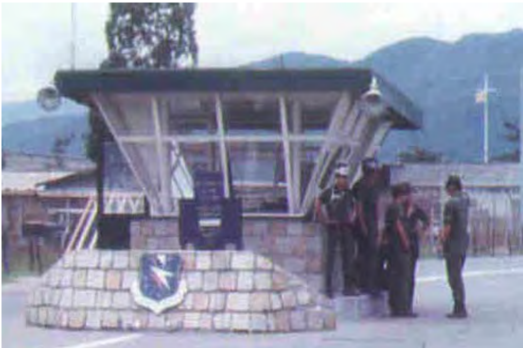
4. Nha Trang AB, Main Gate, close up. SPS. Photo by Domenic Sebben. 1969-1970.
