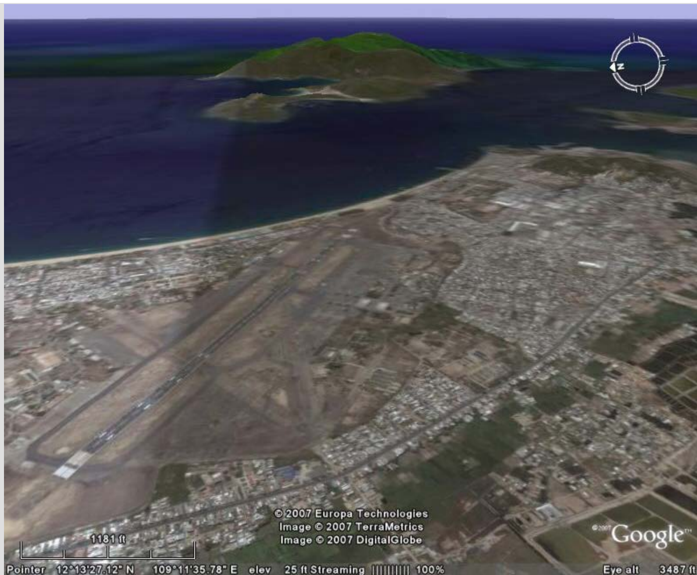
HTI Radar, imaged/angled East at 3,487 feet, as viewed over Nha Trang AB.
