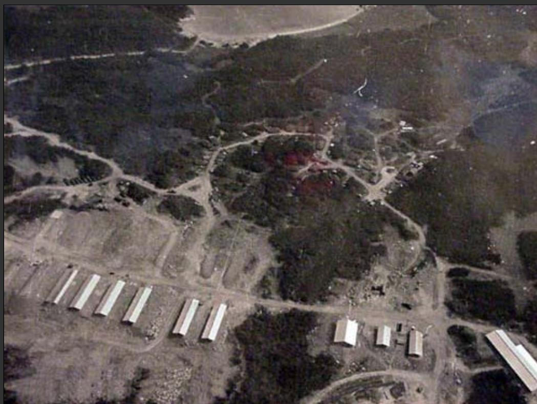
Hon Tre Island, Portcall Radar, Barracks
