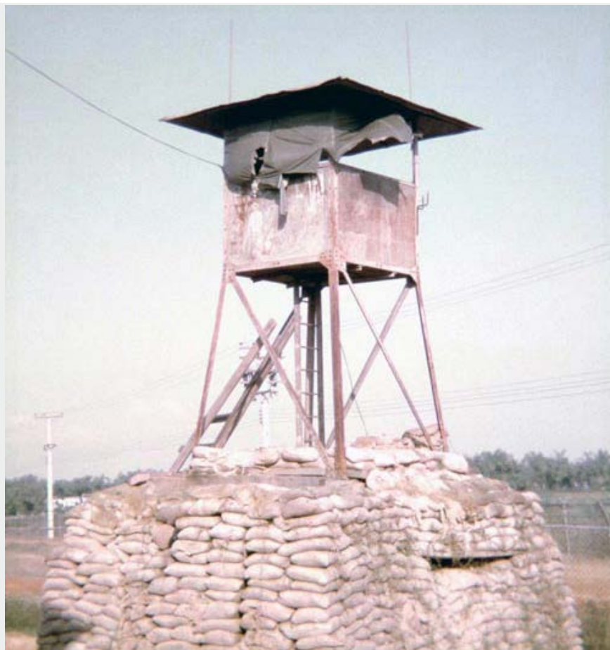
7. Đà Nẵng AB perimeter Bunker and Tower. Photo by Mel Hecker, 1967.
