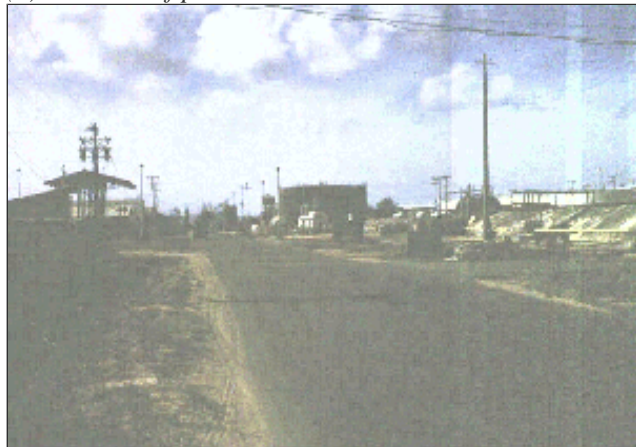
(1) N/B view of perimeter road.
