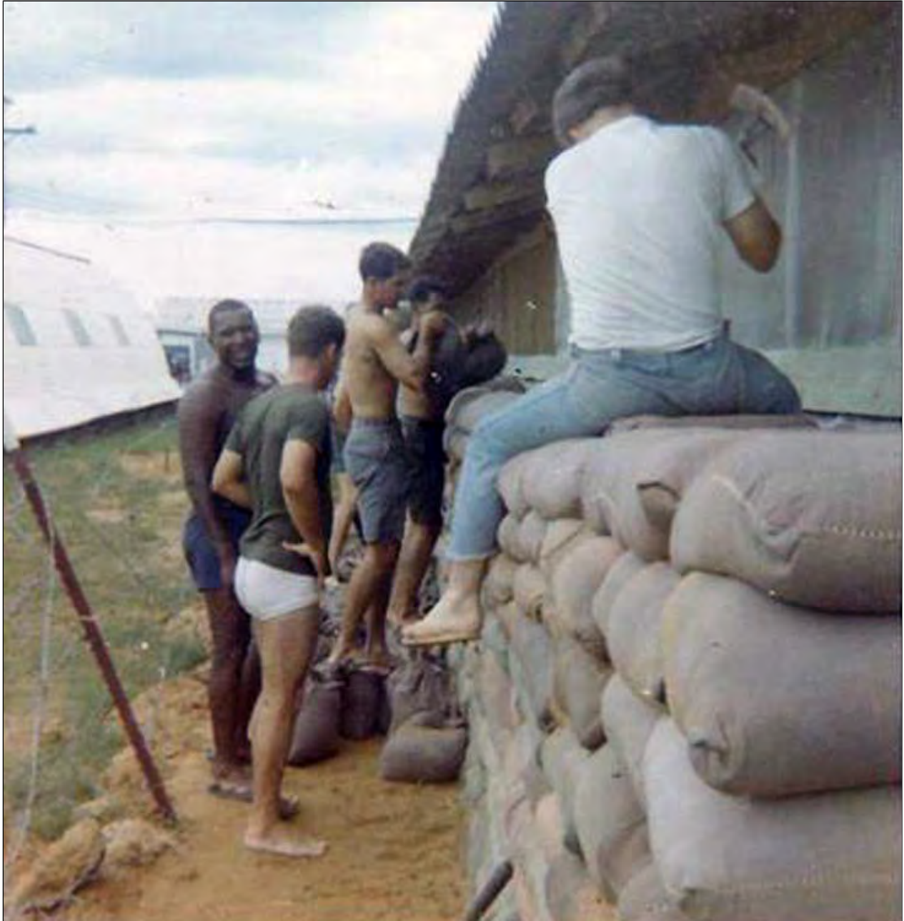
8. Đà Nẵng AB, 366th SPS. Adding layers to sandbag wall around huts. Photo by: Robert A. Lee 1966-1967.
