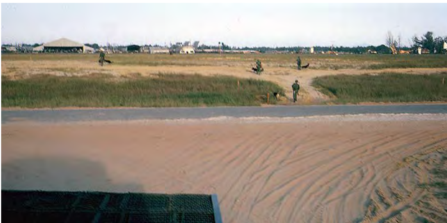
72. Đà Nẵng AB, K-9 Growl Pad: Handlers and Dogs scatter eastward to posts, which could range from 1000-2000 feet long. Across the active runway you can see flight line hangars and buildings. The area immediately in front of the handlers is the under-construction new runway. 1965-1966.
