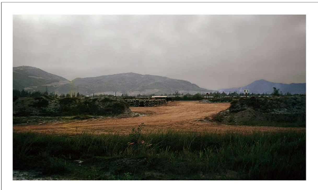
40. Đà Nẵng AB, K-9 Growl Pad: Ammo-Bomb Dump entrance road to Charlie-1 post. 1965.
