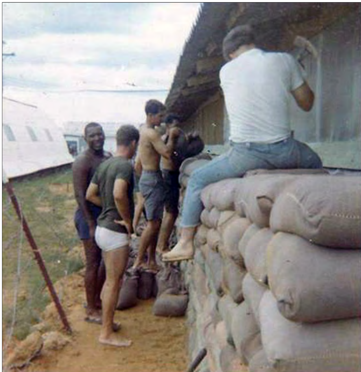
8. Đà Nẵng AB, 366th SPS. Adding layers to sandbag wall around huts. Photo by: Robert A. Lee 1966-1967.
