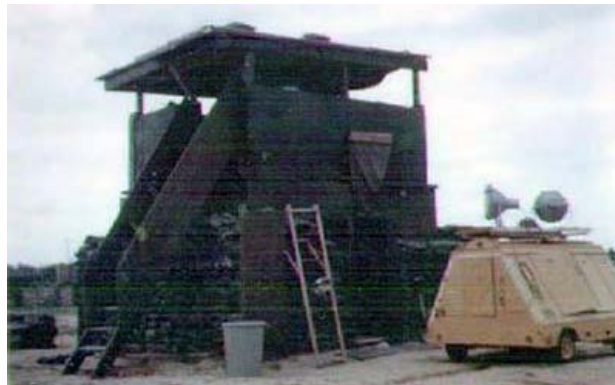
[9] Bunker and tower at the mortar site, south end of Đà Nẵng AB, RVN 1969. Bunker and Tower were used for living quarters for the Mortar Crew, when not on alert or on a fire mission. Was also used as a Fire Direction Control when on a fire mission.
