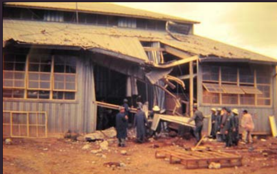
Hangar hit during Jan 3rd rocket attack. 1/68
