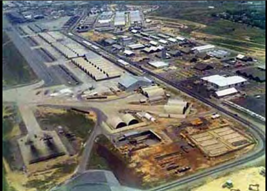
4) S/E end of the runway, Revetment A/C parking in 1966, and hangered by 1970.
