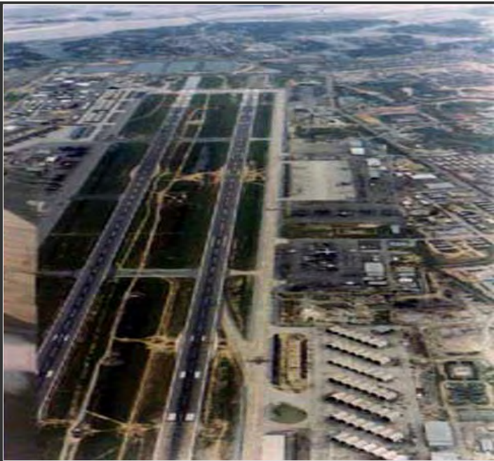
2) Đà Nẵng Air Base runways, 1970.
