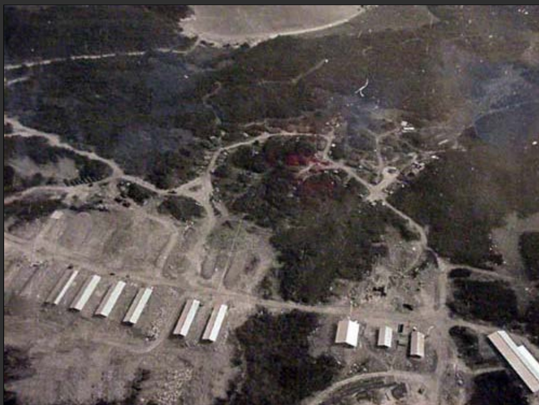
Hon Tre Island, Portcall Radar, Barracks
