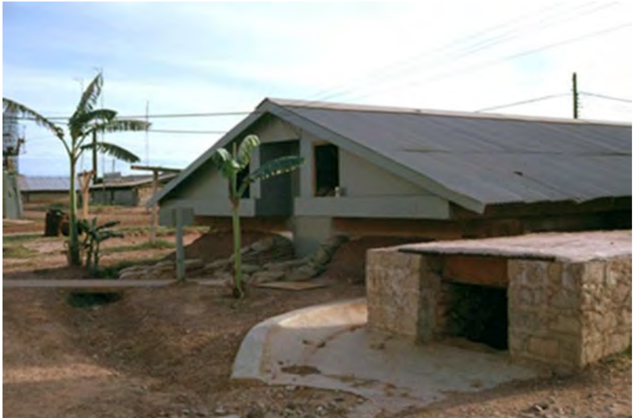
2. Đông Hà Air Field, Admin Hootch and Incoming Rocket/Mortar shelter.
