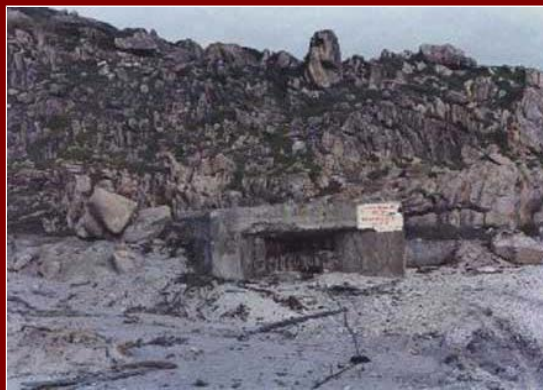
An old French concrete Bunker.
