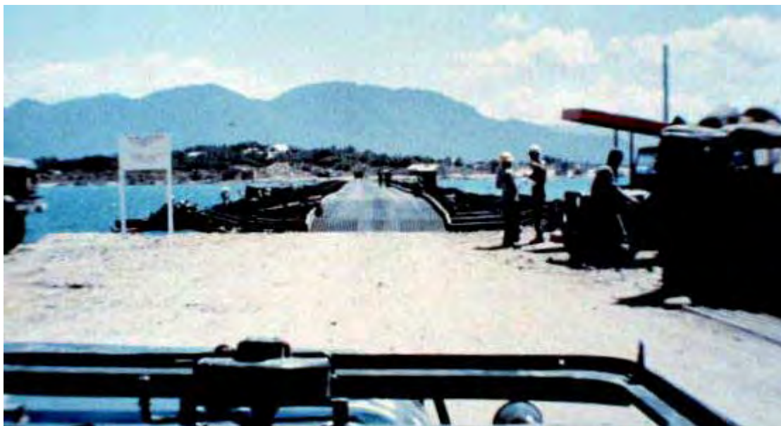
15) Floating Bridge at CRB.
