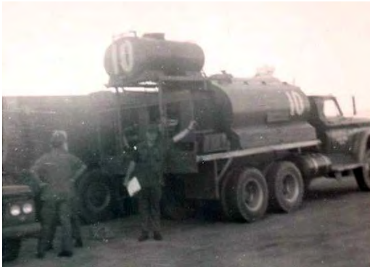
7. We modified a water tanker truck so it could foam the runway.
