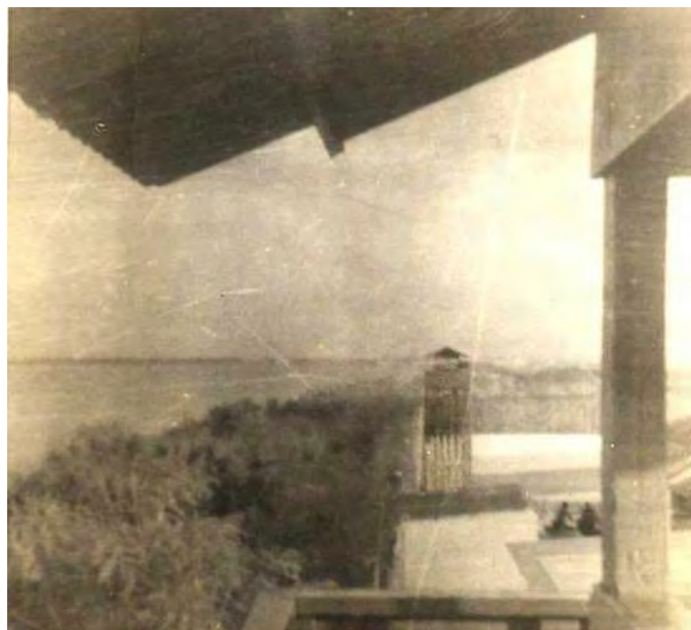
Tower #2 looking at Tower #3 Hilton Compound
