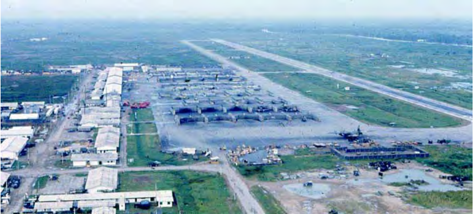
22. Binh Thuy Air Base, Mekong Delta-8 tower, South view. Revetments. MSgt Summerfield, 1968.
