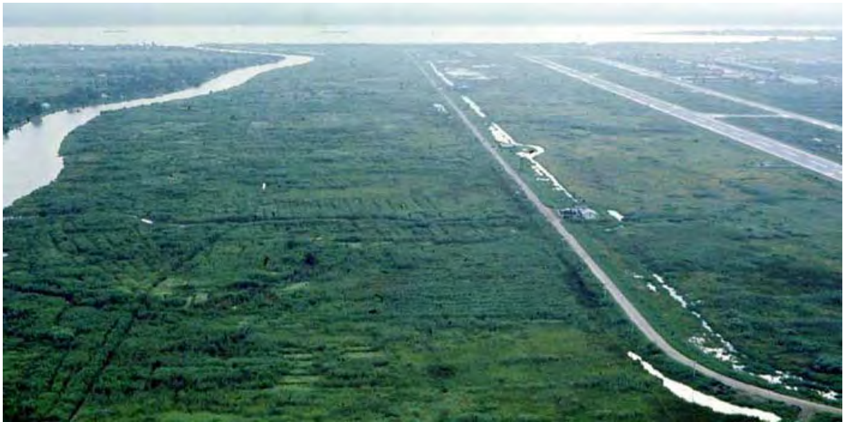
Binh Thuy Air Base, Mekong Delta-1 tower, North view, perimeter towers and bunkers. MSgt Summerfield: 09
