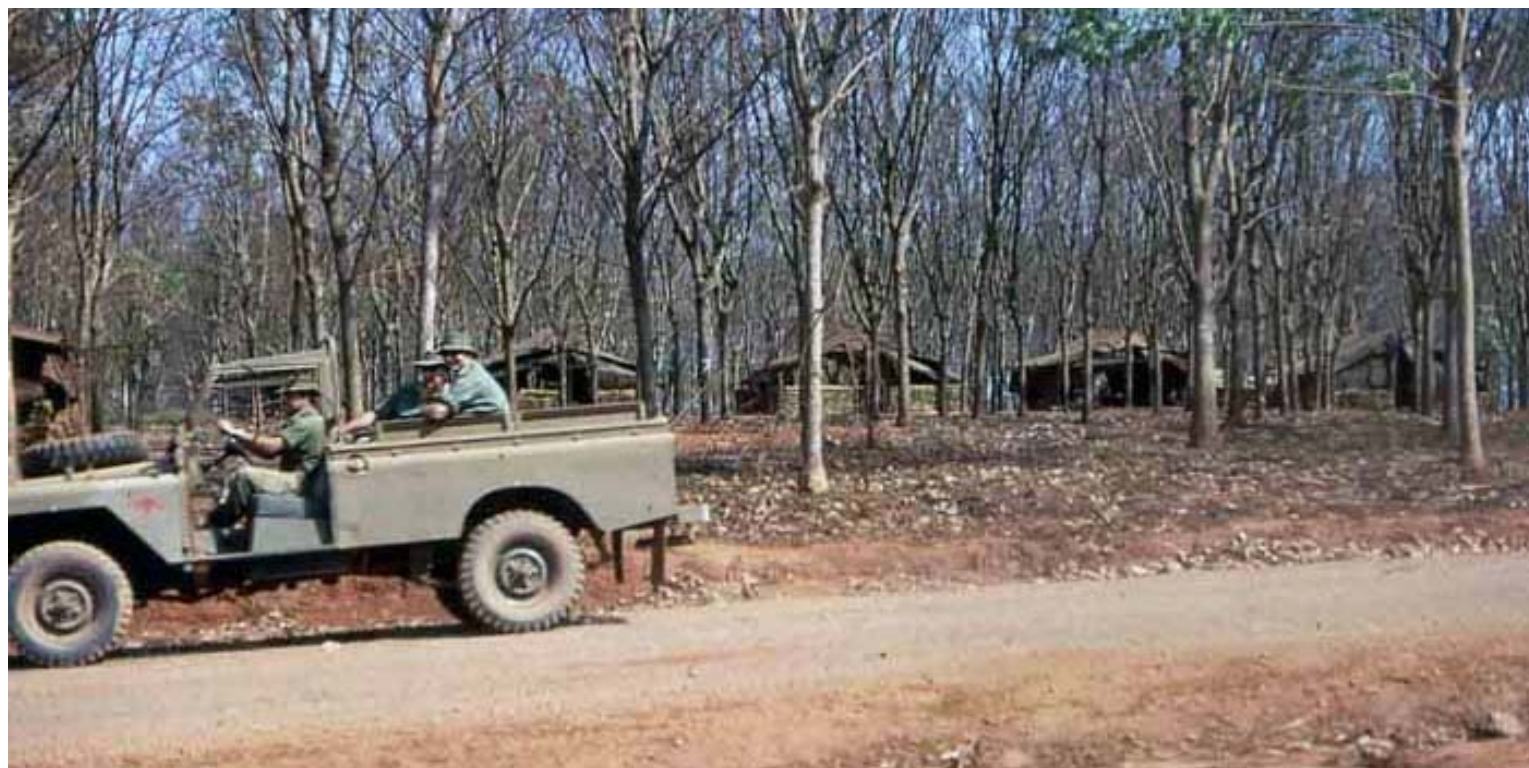
Nui Dat, Australian Artillery Base Housing. MSgt Summerfield: 09
