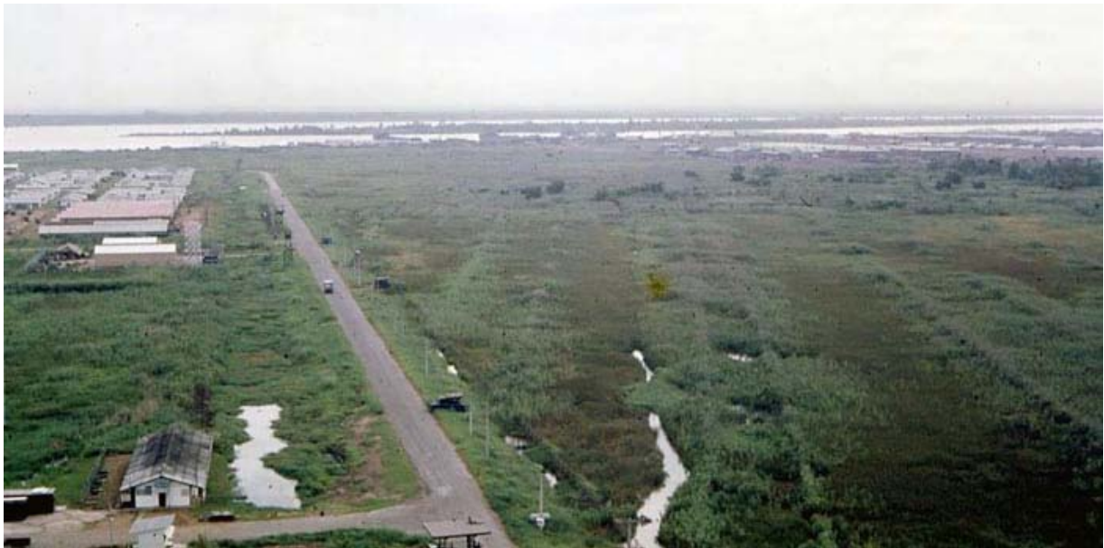
Binh Thuy Airbase, Mekong Delta-3 tower and perimeter bunker. MSgt Summerfield: 14
