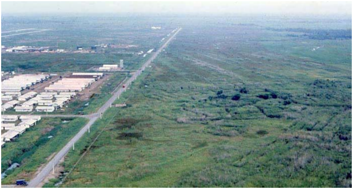
Binh Thuy Airbase, Mekong Delta-4 tower and perimeter bunker. MSgt Summerfield: 13
