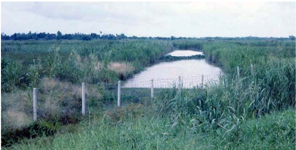
Binh Thuy Airbase, perimeter road flood channel. MSgt Summerfield, 1968: 26
