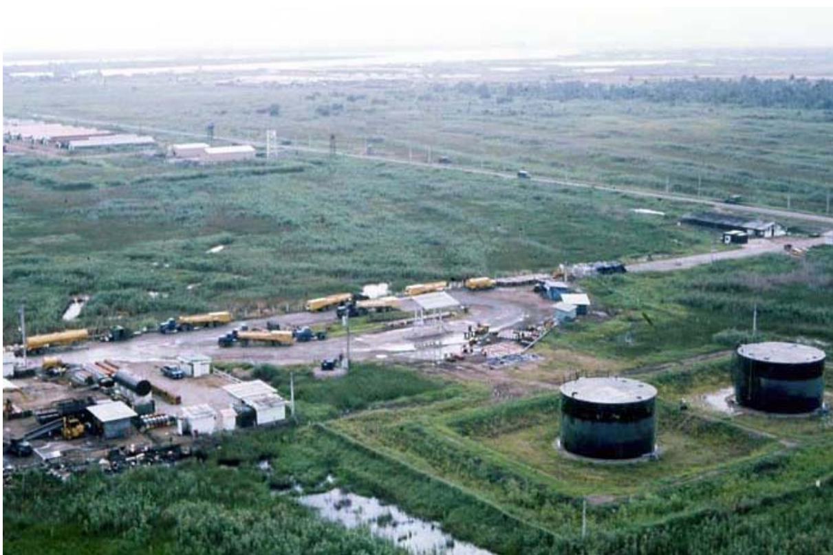
Binh Thuy Airbase, POL tanks and POL canopy pumps that burnt in TET 1968. MSgt Summerfield, 1968: 18
