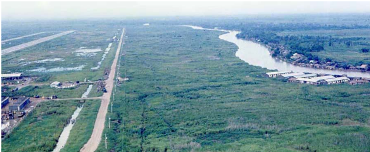
Binh Thuy Airbase, Mekong Delta-5 tower and perimeter bunkers. MSgt Summerfield: 11
