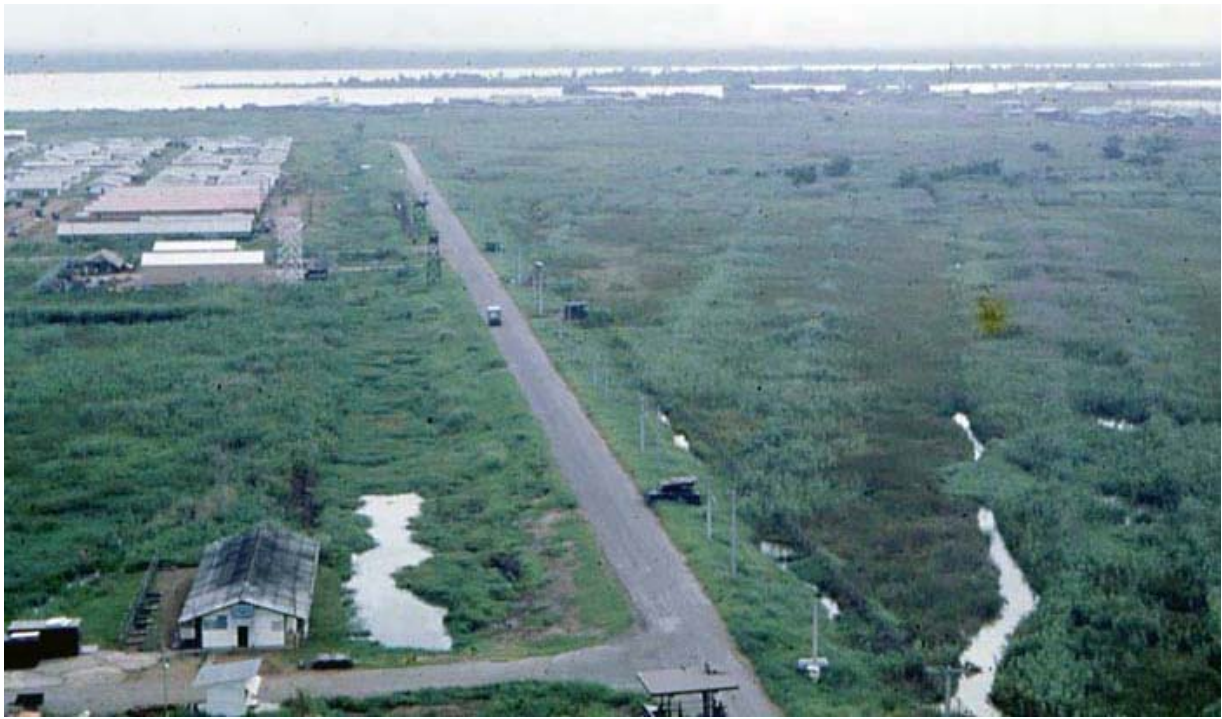
Binh Thuy Airbase, Mekong Delta-3 tower and perimeter bunker. MSgt Summerfield: 15
