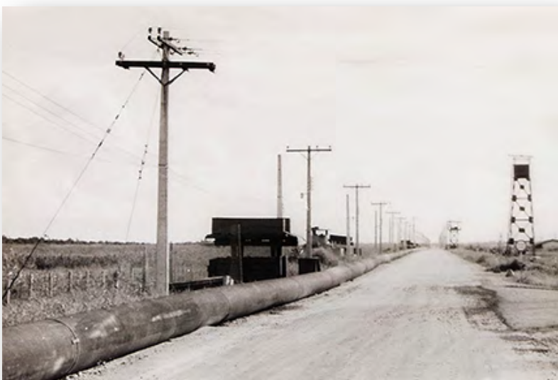
1: Binh Thuy AB: Perimeter, Bunkers and Towers.
