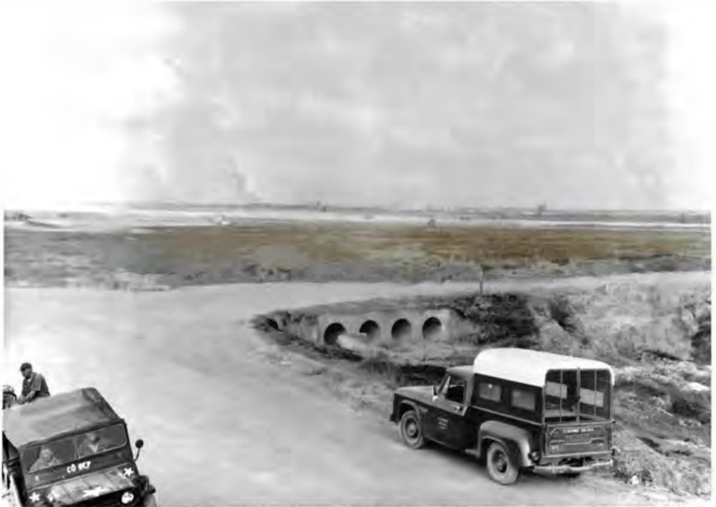
66. Photo Right: Typical perimeter road culvert as seen from Bunker Hill-10.
