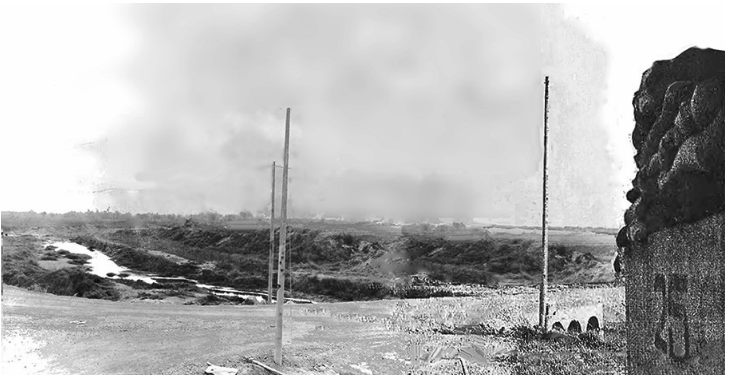
Bunker Hill-10: Perimeter Road. Ditch and culvert under road where VC crossed through.
