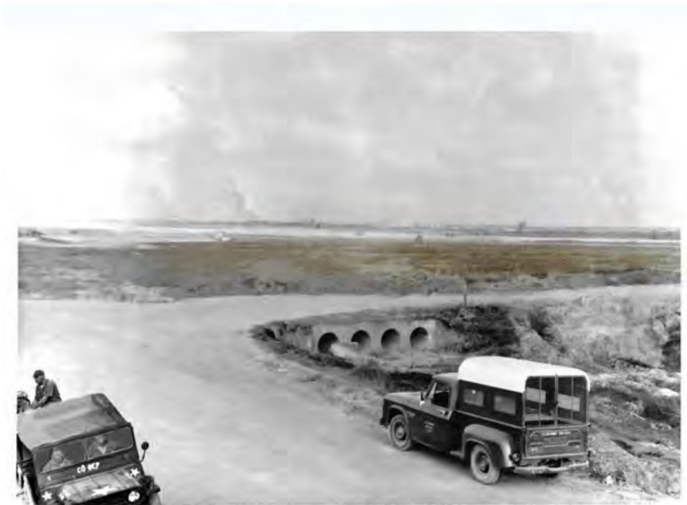
Typical perimeter road culvert as seen from Bunker Hill-10.
