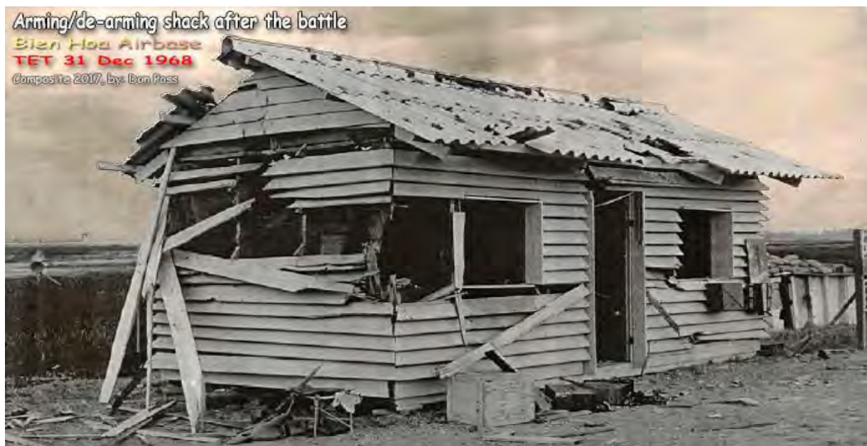
Photos: Biên Hòa Air Base: Aircraft Run-up Arming/de-arming Pad shack.
