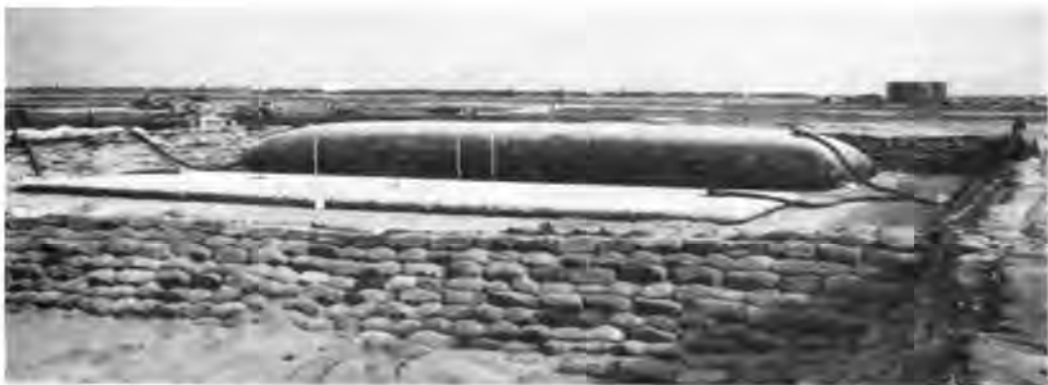
Dikes constructed to protect petroleum supplies at Tuy Hoa Air Base
