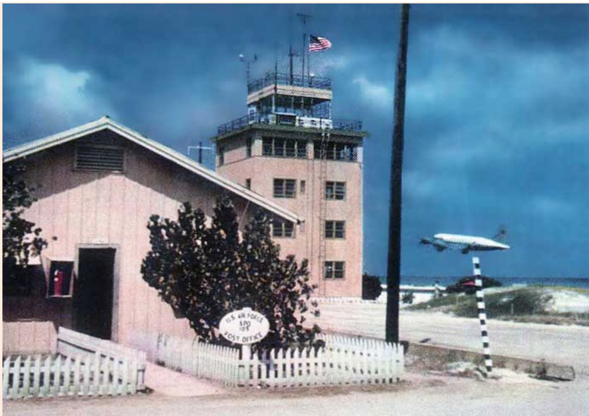
2. Johnston Island, Agent Orange storage. Control Tower and U.S. Post Office.
