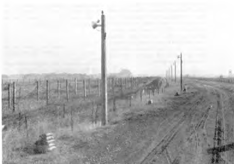
Antipersonnel directional mines installed inside the perimeter fences at Tan Son Nhut Air Base. Sandbags protected defenders from back blast
