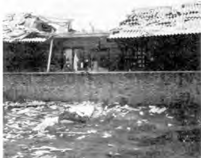
Brick revetments constructed about billets at Pleiku Air Base to protect against shell fragments. Such revetments were useless against direct hits
