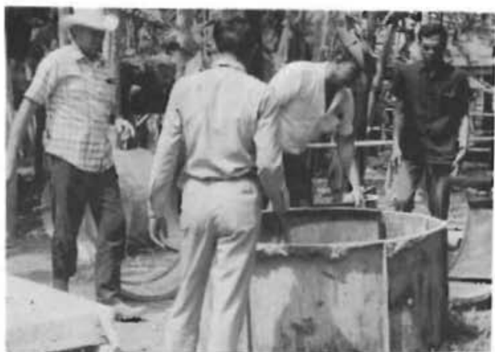
INSTALLING A WELL
