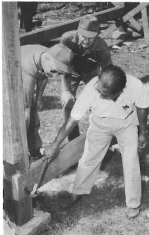
BUILDING A SCHOOL
