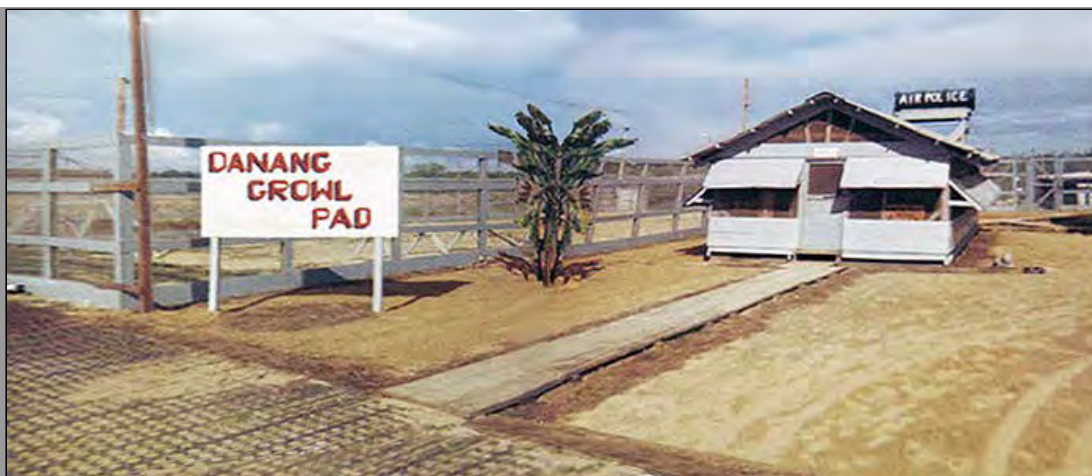
3. Đà Nẵng AB, K-9 Growl Pad: Growl Pad's new office building. 1965.
