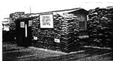
Central Security Control.
