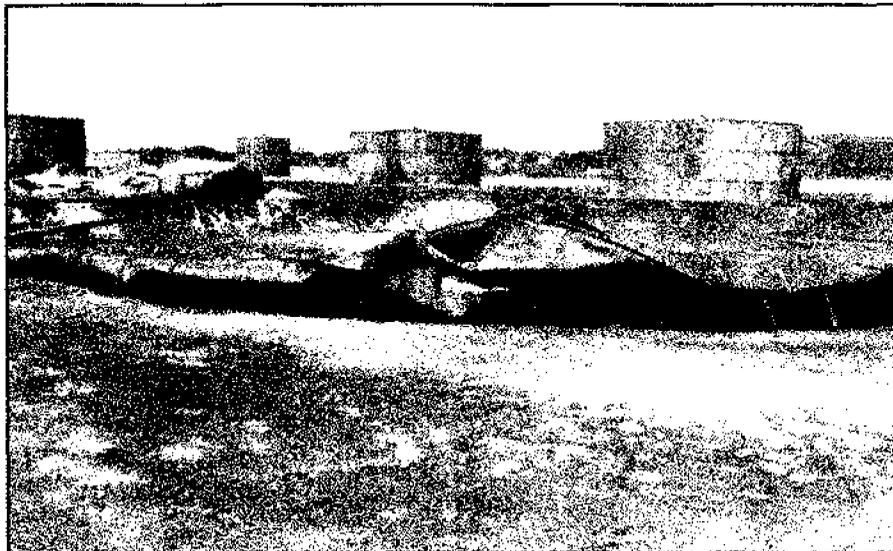
This is the remains of the POL tank involved in the Sapper attack, refer to the story 'Smelling like a Rose' The tanks in the back ground showed effects of the intense heat but did not burn, they were filled with JP4. We were lucky that other tanks did not explode causing more damage. There were satchel charges placed at other tanks but they did not cause the fire this one did.
