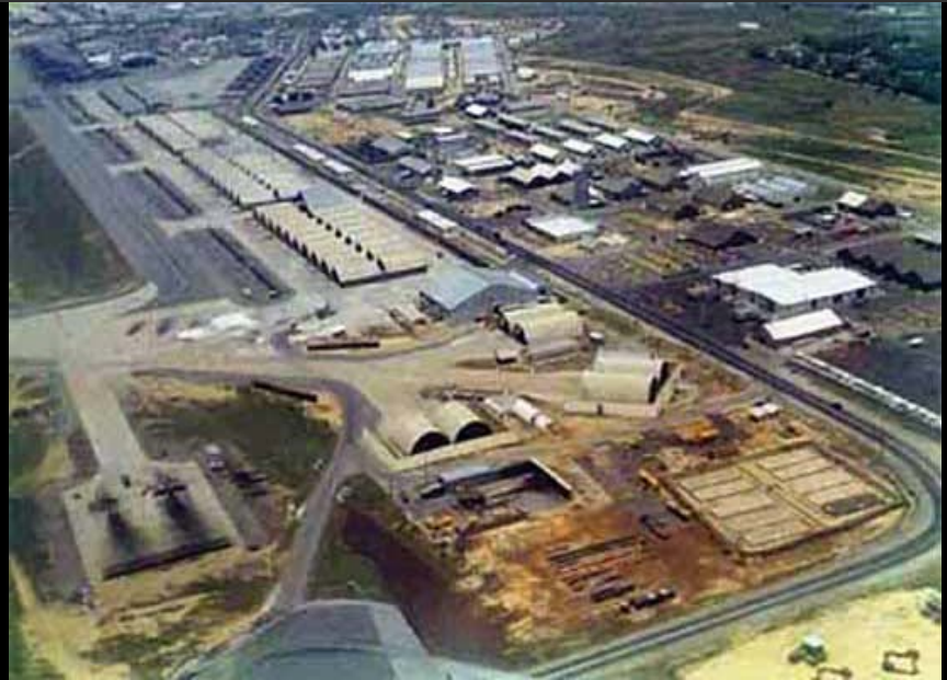
4) S/E end of the runway, Revetment A/C parking in 1966, and hangered by 1970.
