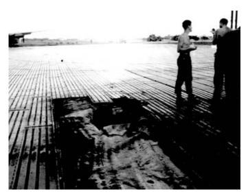
Late 1966, a mortar hit on the aircraft parking area on the north side of runway. The Seabees of my detachment performed the repairs to Dông Hà Air Field's aluminum / magnesium runway matting and the PSP parking area.
