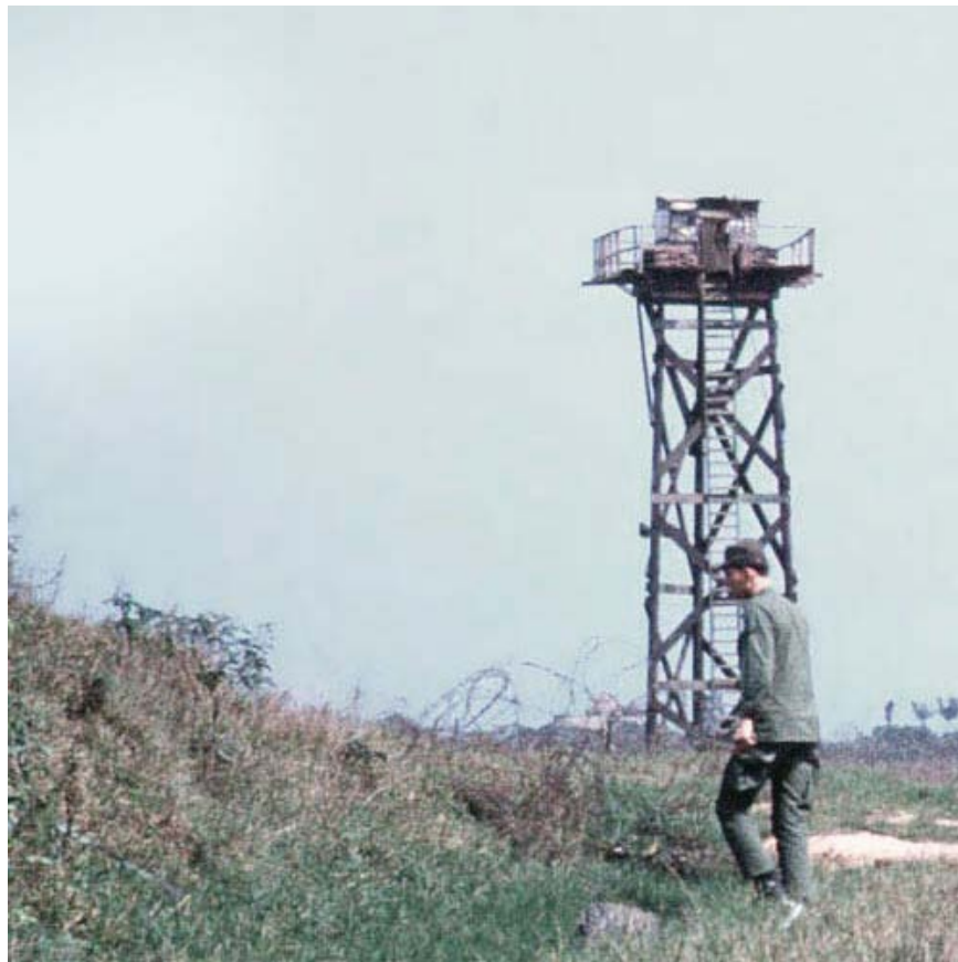
3. Đông Hà Air Field: Close Up, Perimeter and setting Mines.
