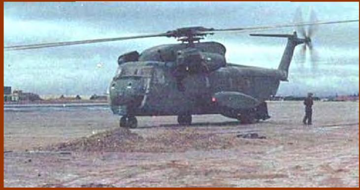
Đông Hà Air Field 1968, Steel runway, with trenches near where aircraft taxi to unload cargo due to being in range of NVA artillery.
