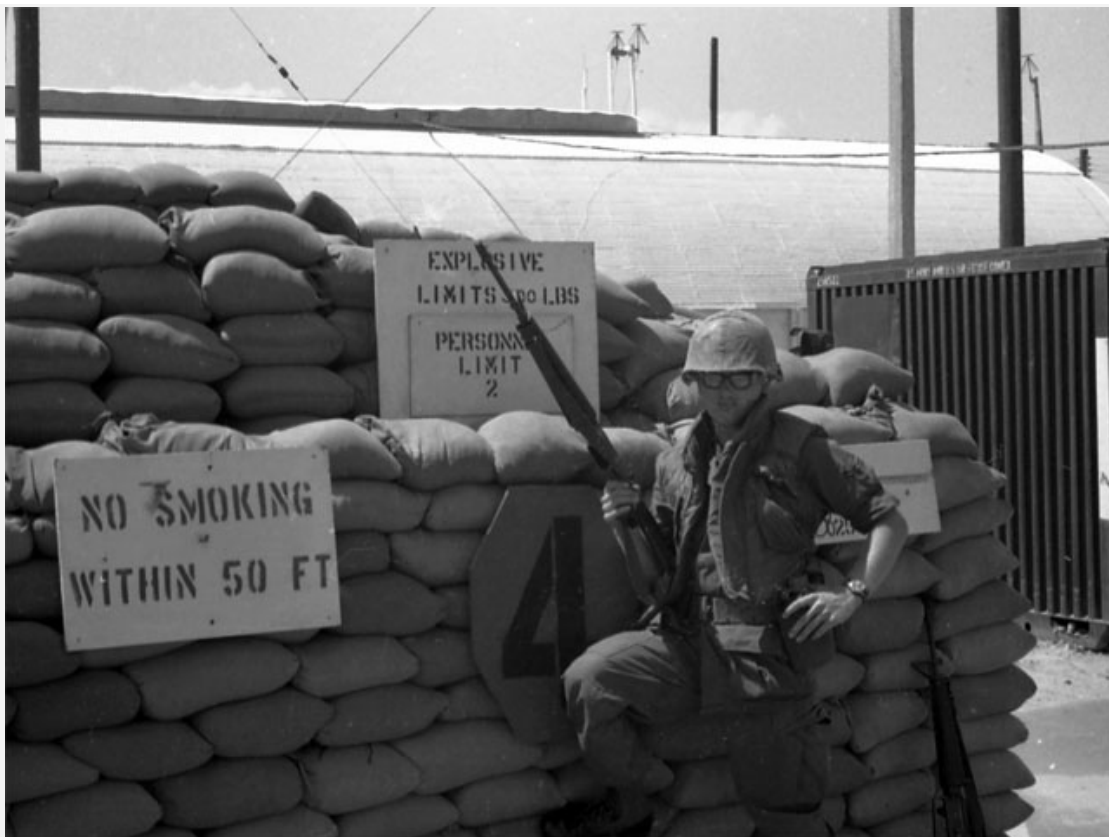
19. Cam Ranh Bay AB, SP Explosives Bunker. 1969-1970.
