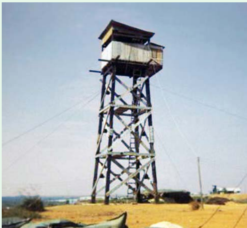
1. Chu Lai AB, Perimeter Tower. Note the tower (lower-right) on horizon. Photo by unknown.
