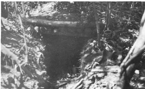
In contrast, a VC bunker built to withstand direct hits from artillery and bombs is extremely well camouflaged.
