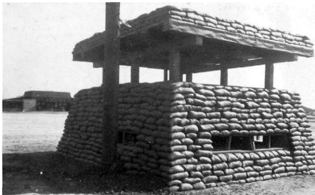
Two approaches to fortifications: an American-built firing bunker defends the vital Long Binh base area, an important target for the Tet Offensive. Such positions were easily plotted by VC recon detachments.
