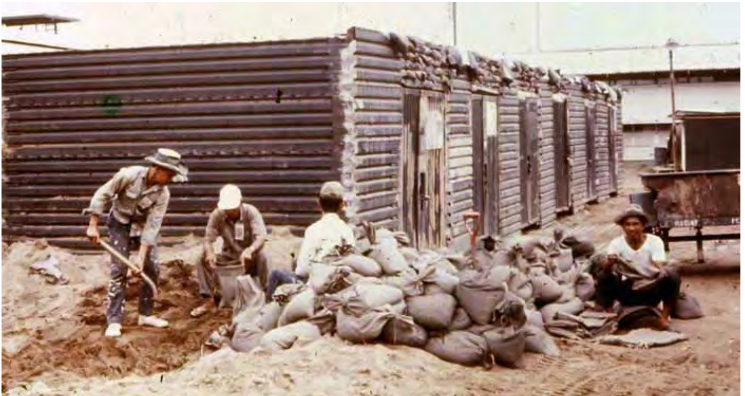
33. Binh Thuy Air Base, Vietnamese workers are either sandbagging , or filling sandbags, during bunker construction next to ammo storage revetments. MSgt Summerfield.
