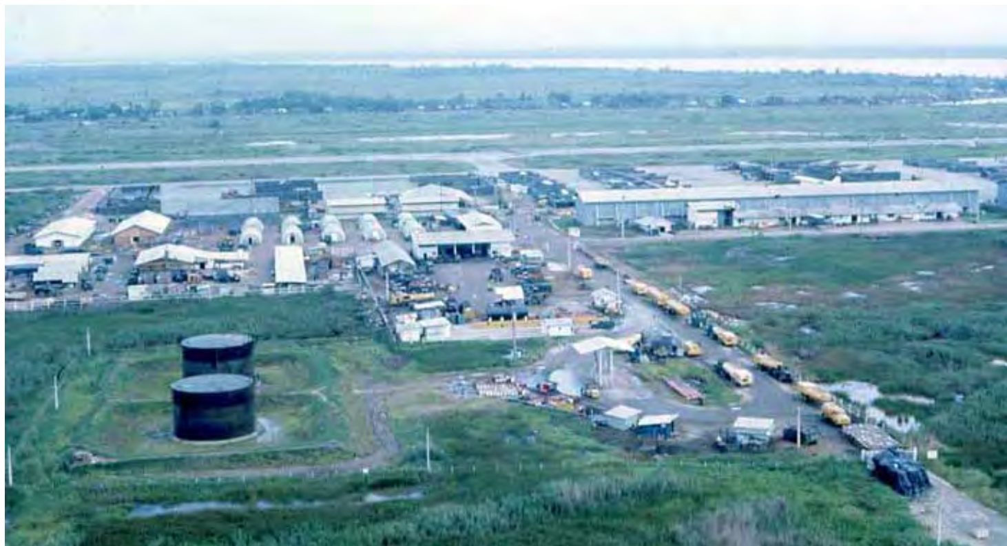
Binh Thuy Air Base, POL tanks and POL canopy pumps that burnt in TET 1968. MSgt Summerfield, 1968: 17
