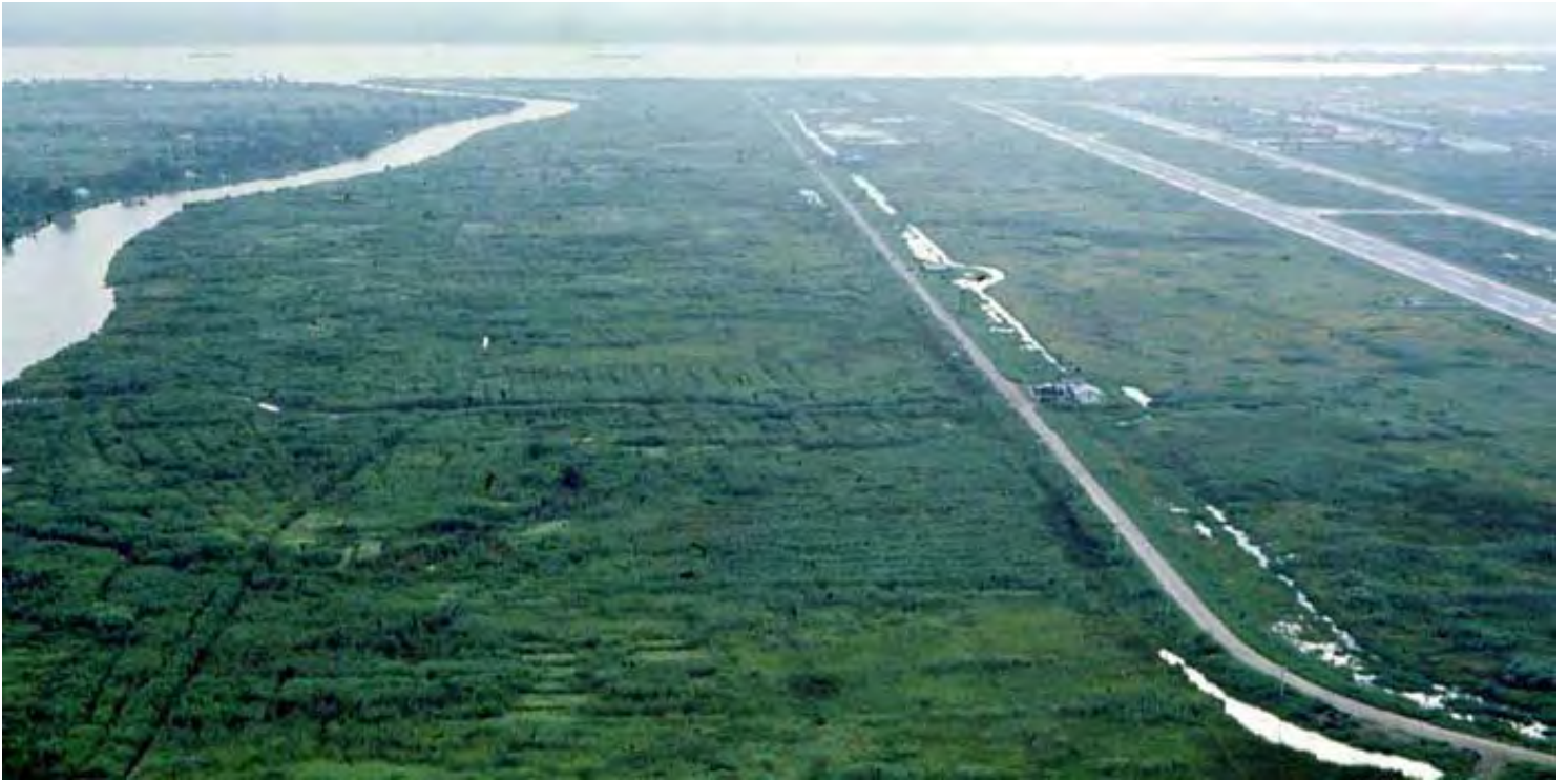
Binh Thuy Air Base, Mekong Delta-1 tower, North view, perimeter towers and bunkers. MSgt Summerfield: 09
