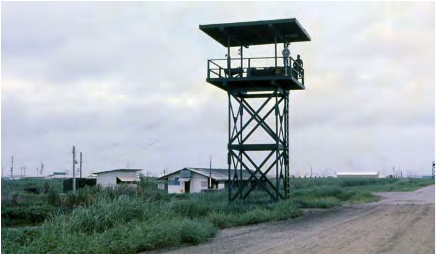
Binh Thuy Air Base, perimeter road SPS Tower. MSgt Summerfield, 1968: 25
