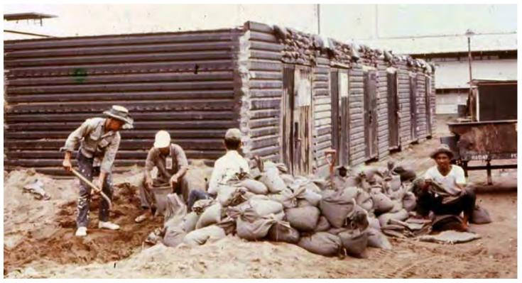
33. Binh Thuy Air Base, Vietnamese workers are either *sandbagging*, or filling sandbags, during bunker construction next to ammo storage revetments. MSgt Summerfield.
