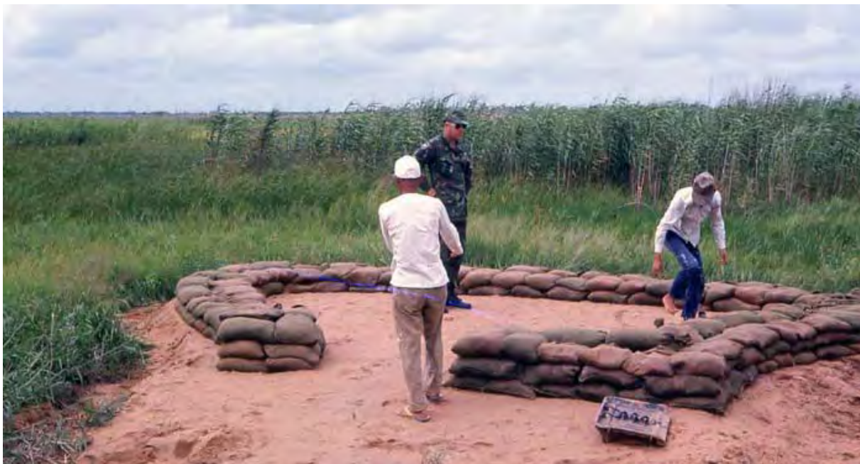
Binh Thuy Air Base, SPS Airman mans instructs Vietnamese workers building Listening Post. MSgt Summerfield: 07 (Good job... see you tonight!)
