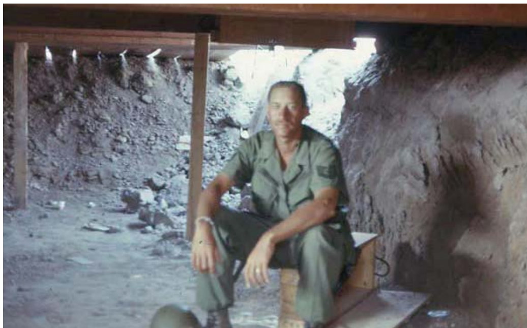
Tân Sơn Nhứt AB, 377th SPS, Bunker outside. MSgt Summerfield: 04
